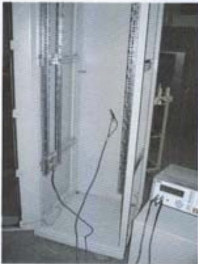
ground continuity between the chassis and the rear panel
