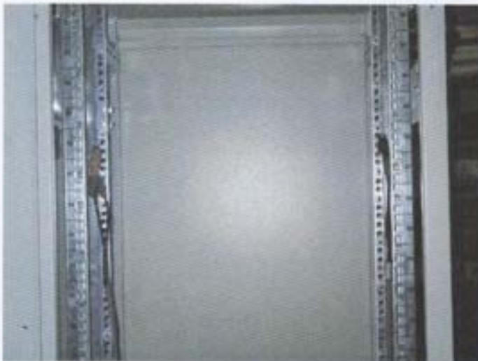
ground continuity between the right and left uprights
