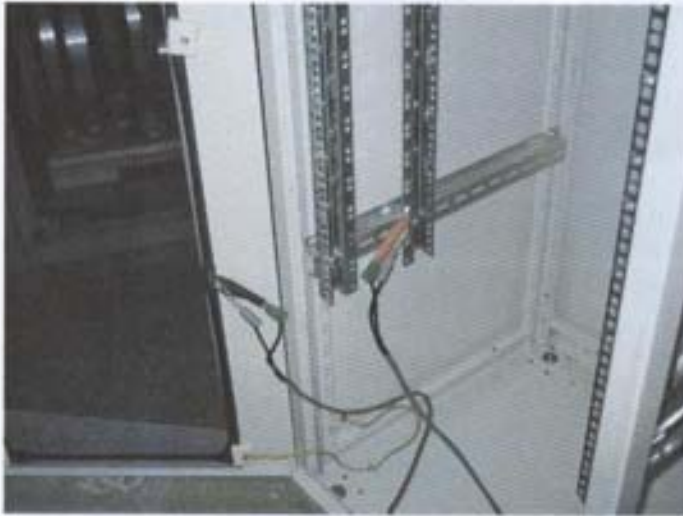
ground continuity between the chassis and the front door
